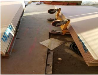
The Telpro Panel lift Plasterboard Cart is an unsafe piece of plant due to instability once they are loaded up.
