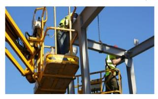
There have been several incidents in Australia and internationally where workers have been crushed against fixed structures while manoeuvring raised boom and scissor type elevating work platforms (MEWPs). Many of these incidents have resulted in fatalities.
