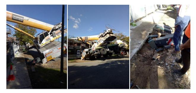
Following an incident on Monday 26/06/2017 where a slewing mobile crane tipped over due to an out rigger breaking through a water pipe the CFMEU recommend the following when setting up mobile cranes and truck mounted concrete placing booms:
