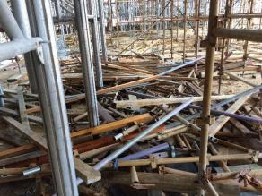
This action is clearly in breach of Regulation 3.81 (2) of the Occupational Health & Safety Regulations 1996. The dropping of this material is clearly in breach of Regulations and must not be done. Proper tools in the form of claw hammer, pinch bar and cold chisel are to be used. Props are only to be used for the purpose for which they are designed, e.g., as adjustable props, not as levers.
