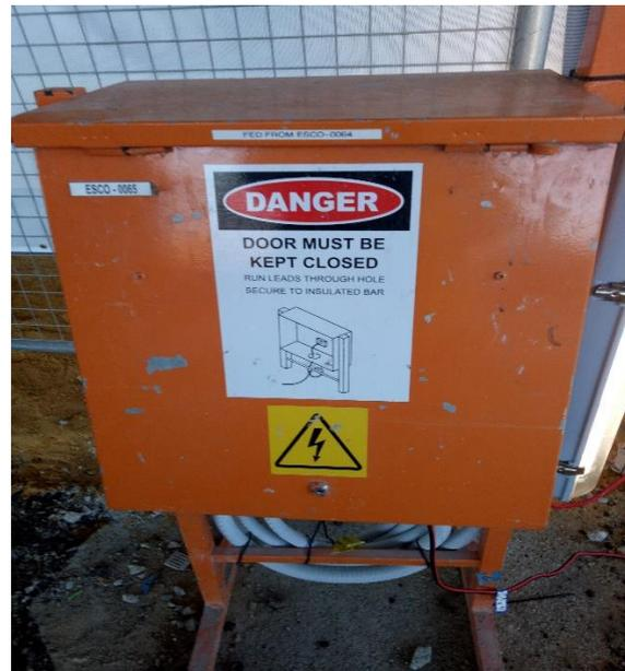
**Testing and tagging** all (PEE) must be tested and tagged every 3 months by a trained competent person. PEE to be tested includes, power tools, flexible leads, lead extension sets, portable DB's & RCD's. RCD's on welding units and EWP's must also be inspected tested and tagged.
