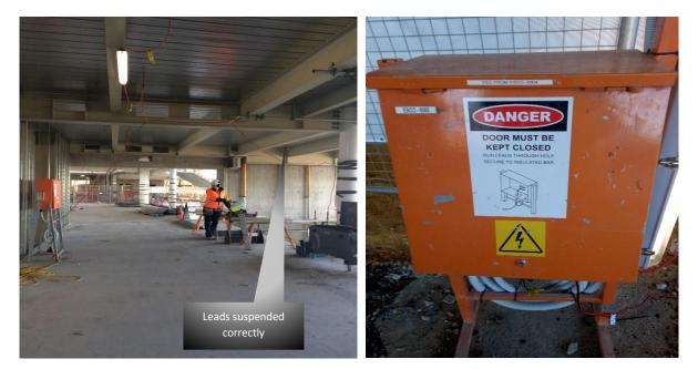
**Testing and tagging** all (PEE) must be tested and tagged every 3 months by a trained competent person. PEE to be tested includes, power tools, flexible leads, lead extension sets, portable DB's & RCD's. RCD's on welding units and EWP's must also be inspected tested and tagged.
